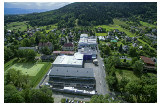
Buczkowice – production & warehouse
